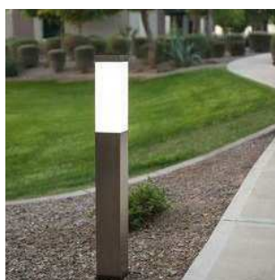
10. NEW BOLLARD WITH LIGHT
